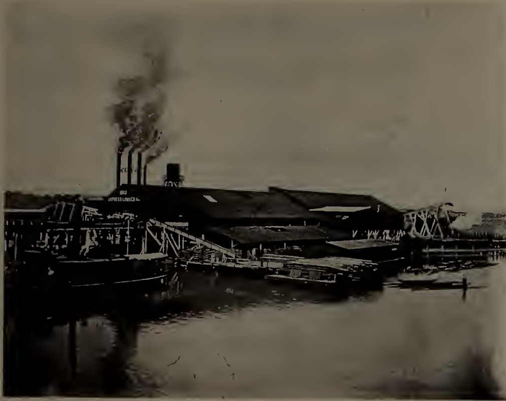
CYPRESS LUMBER COMPANY, 70 Kilby Street. Saw-mill at Apalachicola, Fla.
